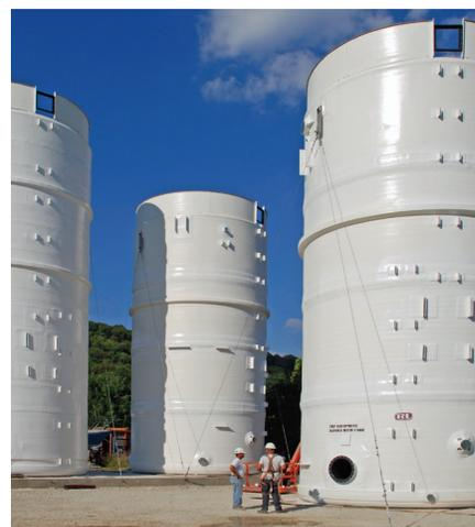
*Tank sections manufactured under ASME-certified conditions were assembled at a riverside site.*
