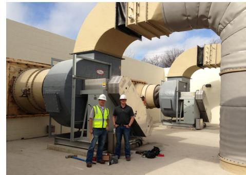
*ECS field service technician Phillip Johnson, left, assists in the start-up, balancing and training of the biofiltration unit.*
