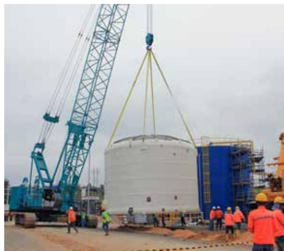
*The manufactured storage vessel is set into place.*
