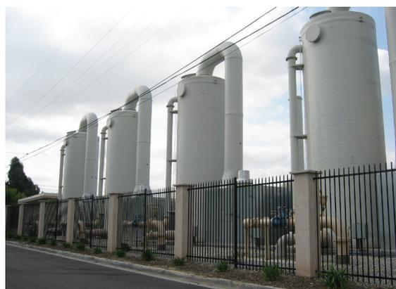
*Air Chem Systems used Vipel® K022-C FR vinyl ester from AOC to manufacture four vertical scrubbers at a water treatment facility in Baldwin Park, California.*
