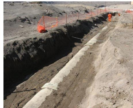
*The project to expand the potable water supply for Arequipa City uses 9.8 kilometers (6.1 miles) of composite pipe.*
