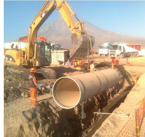
*The lightweight of Flowtite™ composite pipe allowed the pipe to be installed without the use of heavy cranes.*
