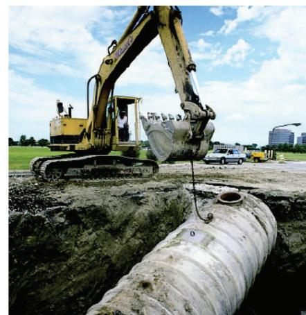
The composite fuel tank was buried under a service station in 1965. The AOC isophthalic polyester was the first to achieve Underwriters Laboratory recognition for corrosion resistance and structural integrity.
