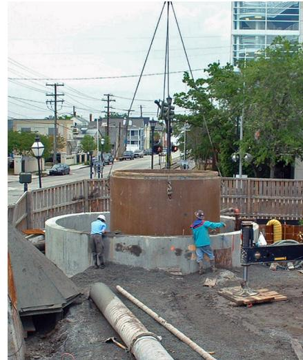
*The huge polymer concrete structures were installed in "stack-up" sections.*
