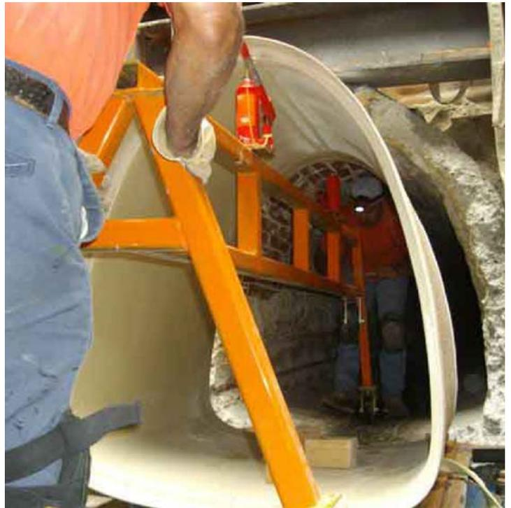
*The original concrete pipe was in danger of failure because much of its protective tile liner was missing.*
