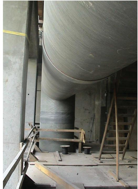
Through its Plastics division, the JTI Companies, Inc., turned to the vinyl ester resin technology and service of AOC to help build a durable new odor control ducting system. JTI provided the detail design, support system engineering and composite cylinders and fittings for a new duct system.
