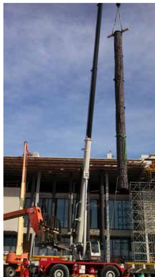
*Installation of the hanging gardens, featuring 67 fiberglass tubes like the one shown here.*
