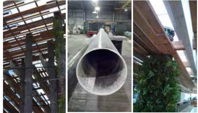
with felt that has pockets cut into it. The plants are placed in those pockets, and water is delivered into the felt through nozzles at the top of the tubes. The water works its way down the tubes, sustaining the plant roots in a soil-less system.
